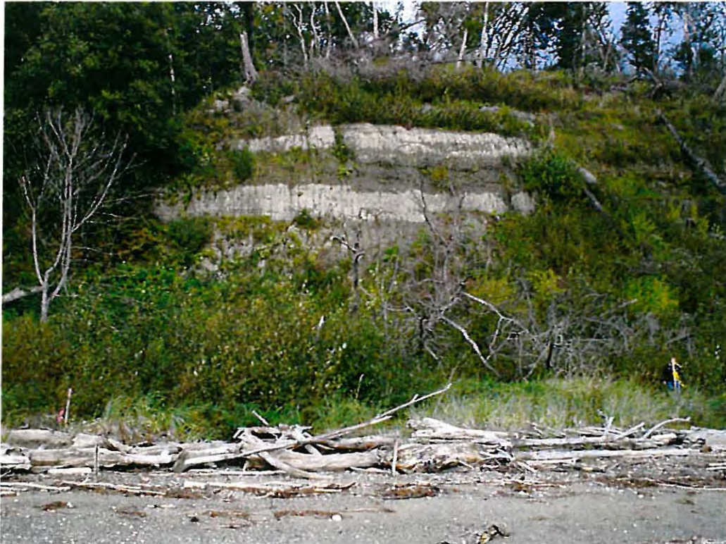
Photograph 1 – View from beach toward upper shoreline at approximate location of conveyor crossing.
